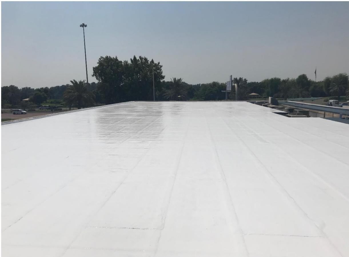
*Liquid Silicone applied on roof top of ADNOC gas station in Abu Dhabi*
